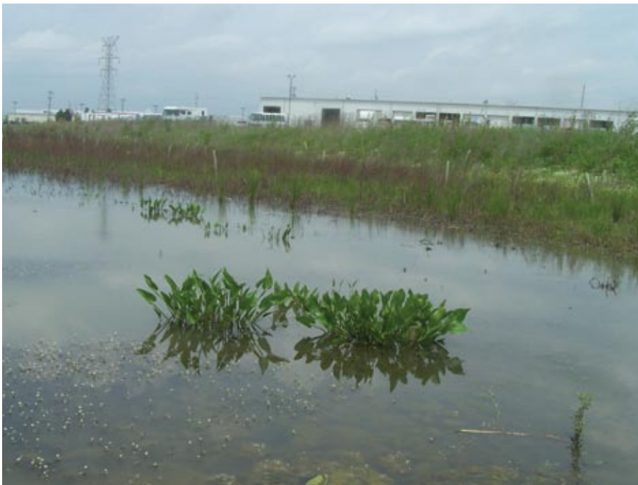
The bioretention ponds are functioning as expected. Post-construction water-quality monitoring has begun, and vegetative survival is also being monitored.
